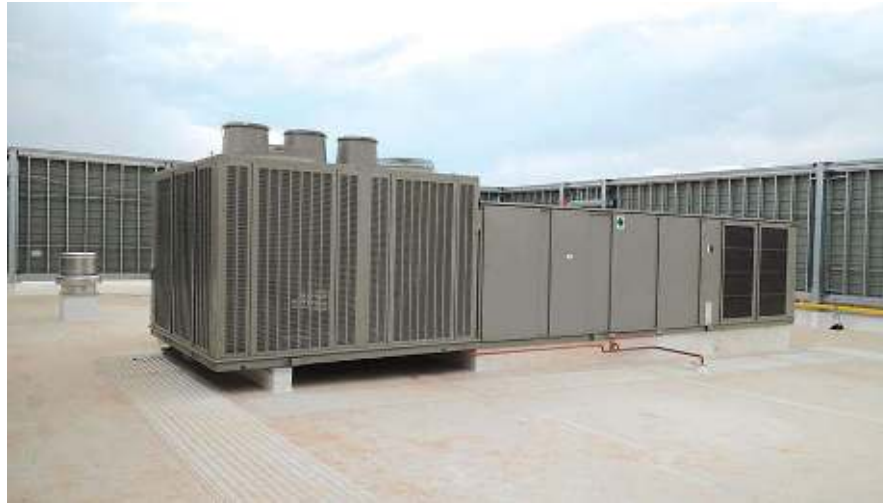
Figure 3: An air-cooled package rooftop unit shows lab exhaust stacks in the background. Courtesy: SmithGroup
