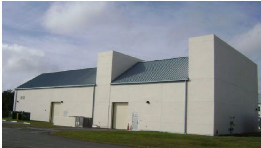
Figure 4: The exterior of an electrical and generator building with intake and exhaust plenums is shown. Courtesy: CDM Smith
