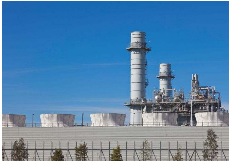
Mechanical evaporative systems are often more efficient than dry systems, reducing water usage at power plants.
