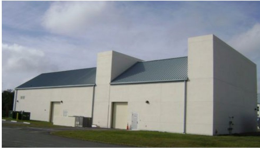
Figure 4: The exterior of an electrical and generator building with intake and exhaust plenums is shown. Courtesy: CDM Smith
