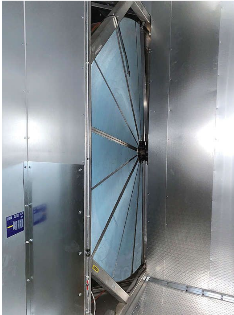
Figure 1: A total enthalpy wheel installed rooftop unit can provide additional energy savings. Courtesy: SmithGroup
