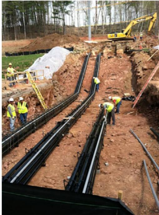
*Electrical conduit provides additional protection for cables in industrial construction projects.*
